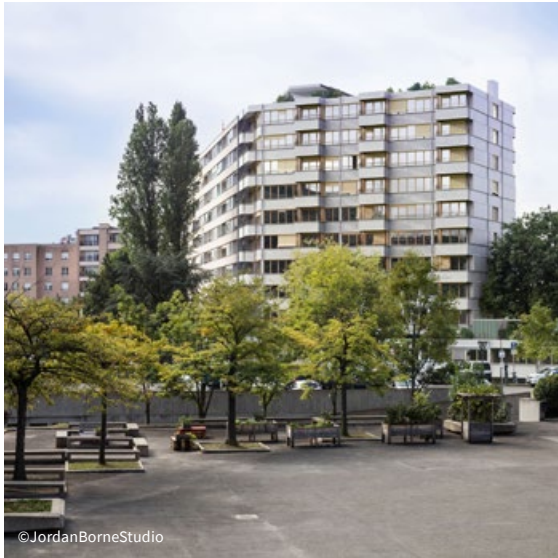
Rue du Valais, Geneva: Development and expansion of mixed-use office premises with small urban apartments
