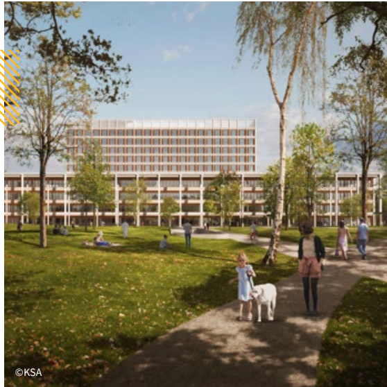
Cantonal Hospital Aarau: Construction of new hospital building as total contractor
