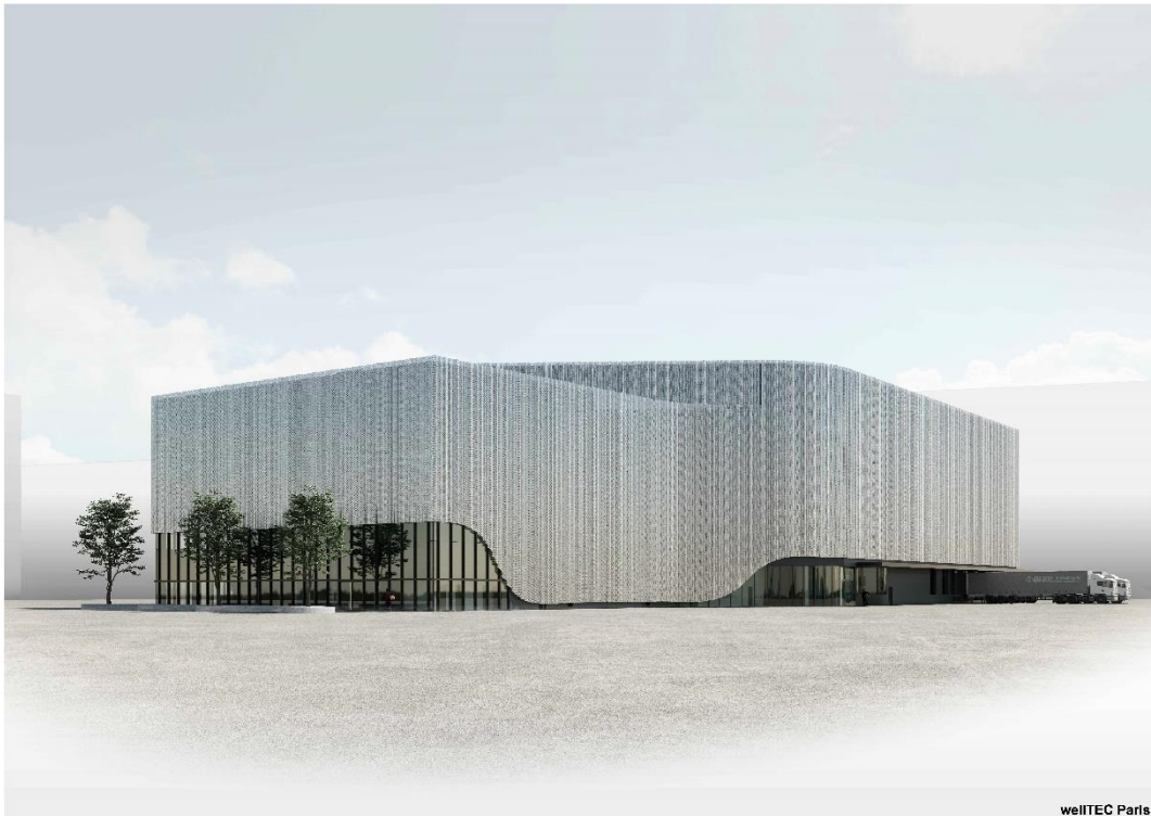
New logistics centre for the USB near the harbour in the Sternenfeld district of Birsfelden (image: ©Burckhardt).
