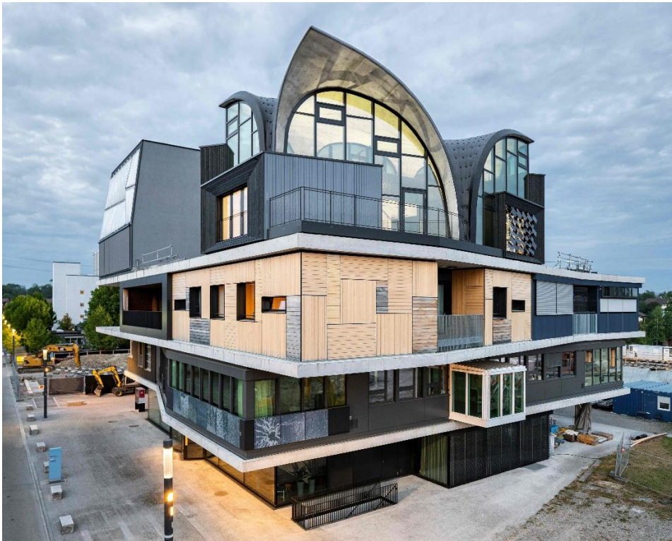
NEST platform at Empa: The new "Beyond Zero" unit will be built on the centre platform of the NEST building (image: ©Roman Keller).
